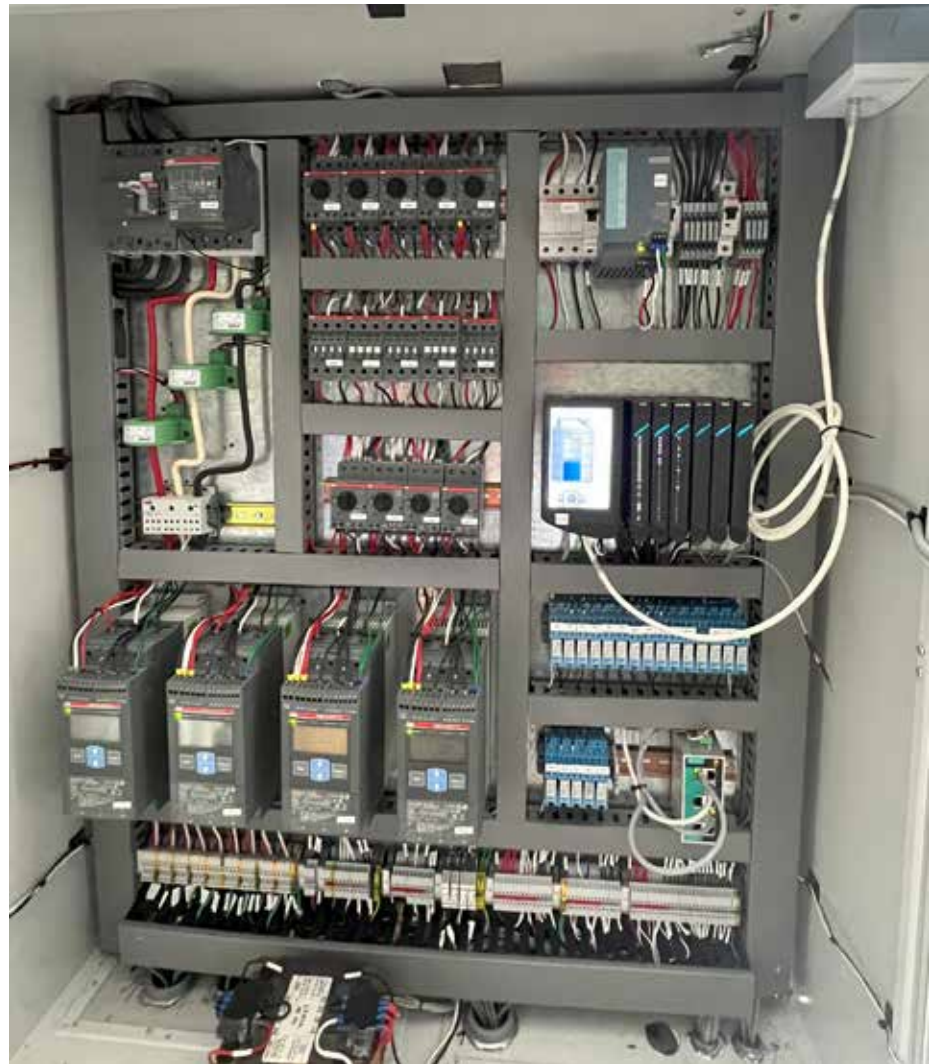
The groov EPIC system (center right) offers a wide -20 to 70 °C operating temperature range.
