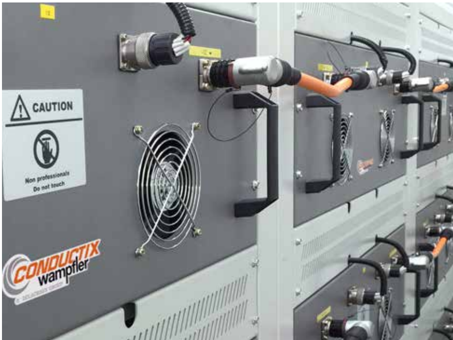
The heart of the Power Packs are lithium-ion batteries of the latest technology in combination with a special battery management system.
