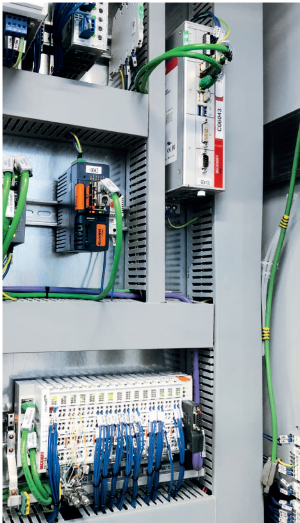
The individual processes within the Aida press lines are controlled by an Industrial PC with TwinCAT software as well as various EtherCAT terminals.
