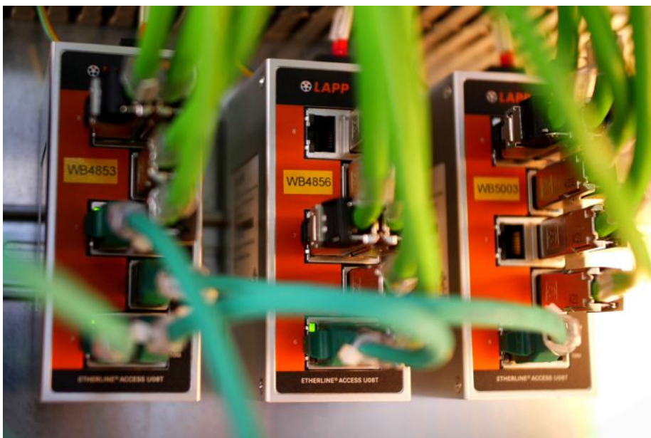
In addition to numerous LAPP data lines and power cables, ETHERLINE ACCESS switches were also used.
